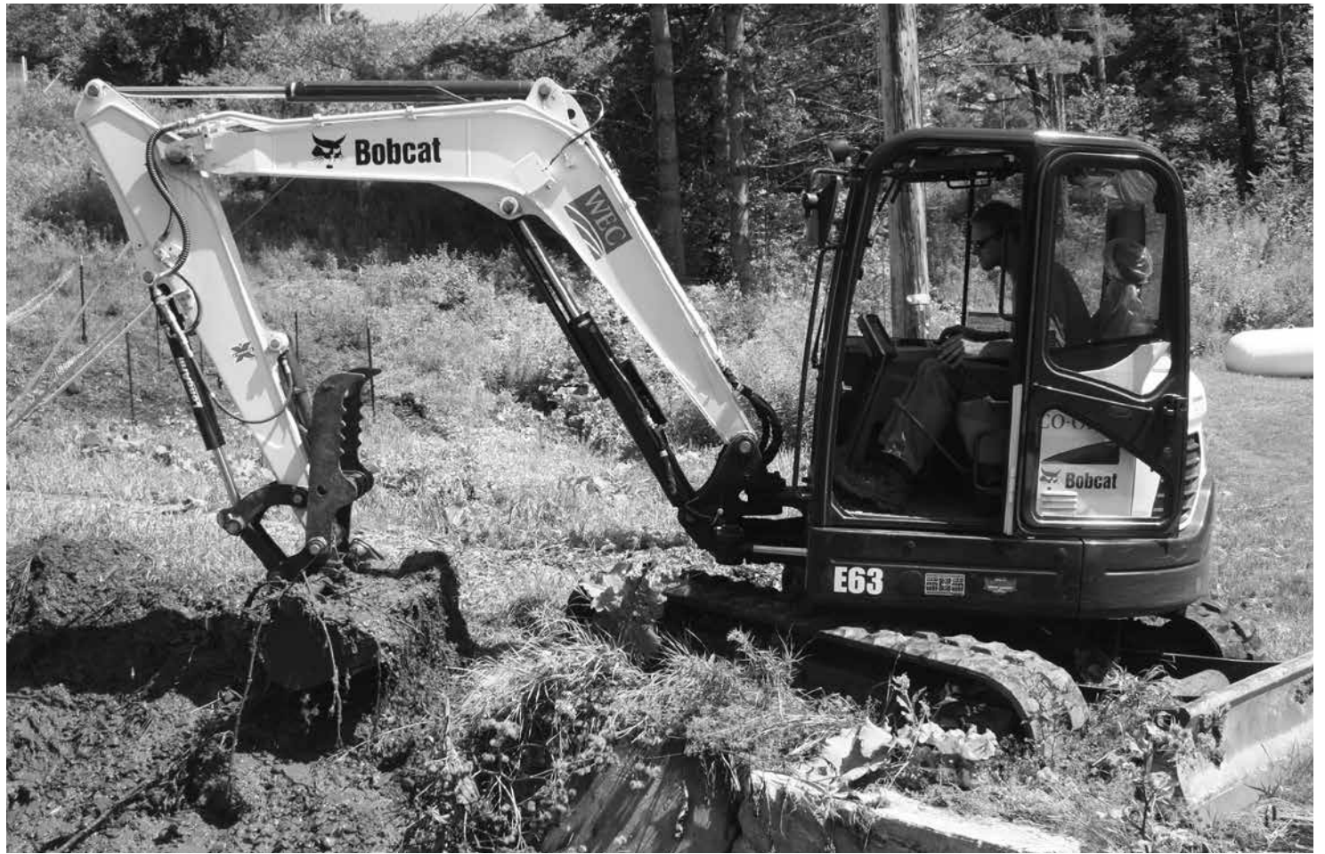
The new eight-ton Bobcat excavator has more than proved its worth since the Co-op purchased it in May. Its compact size, off-road capabilities, and versatility have enabled WEC to keep more of its projects "in-house," and get jobs done more quickly. A feature that gets lots of attention is the Bobcat's "thumb," which it uses to grasp and carry heavy objects.
