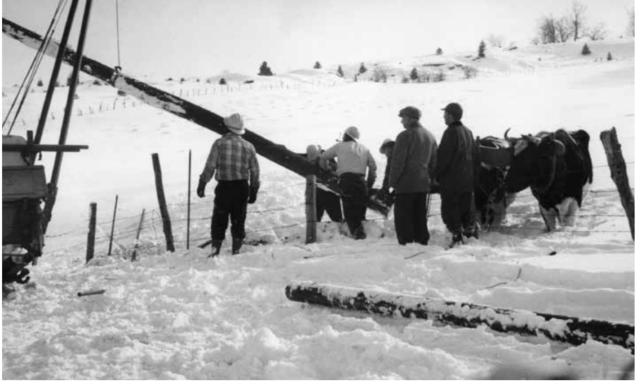
A team of oxen stands ready to assist as men set a power pole during Washington Electric Co-op's early days. Though a truck can be seen on the left, it's likely, because of REA rules, that this section of line then marched off into the countryside. Many of the original rights-of-way are now very difficult to reach and service.
