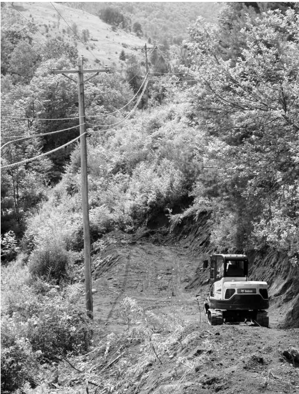
While most right-of-way maintenance consists of routine re-clearing and trimming of vegetation, WEC's history as a very rural co-op means there are areas requiring more extensive work to make them reachable for linemen. An example is this steep, wooded hillside in Chelsea (left). In all projects, WEC follows a vegetation-management plan approved, for any environmental impacts, by state regulators. The equipment works around important vegetation, such as the apple tree in an isolated part of East Montpelier (above), and never disturbs wetlands. All areas are re-seeded with grass immediately after the work, and WEC does not use herbicides in its rights-of-way. At right, Donnie Singleton is seen against the sky atop a steep hill in the almost hidden right-of-way in East Montpelier.
