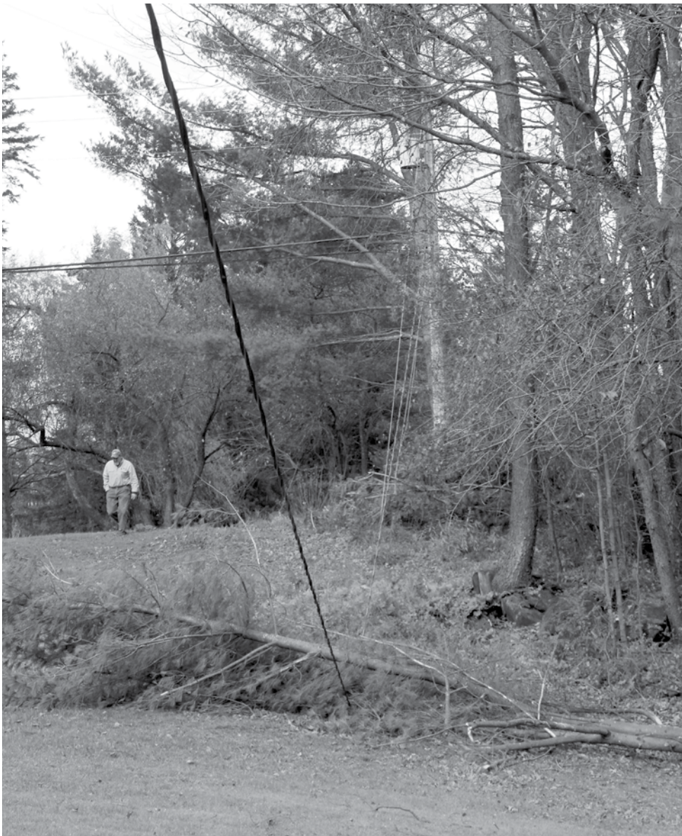
Below: Dan Couture, System Maintenance Technician, on Snow Hill Road in East Montpelier. Crews saw scenes like this throughout WEC's service area: wires pinned to the ground by fallen limbs.
