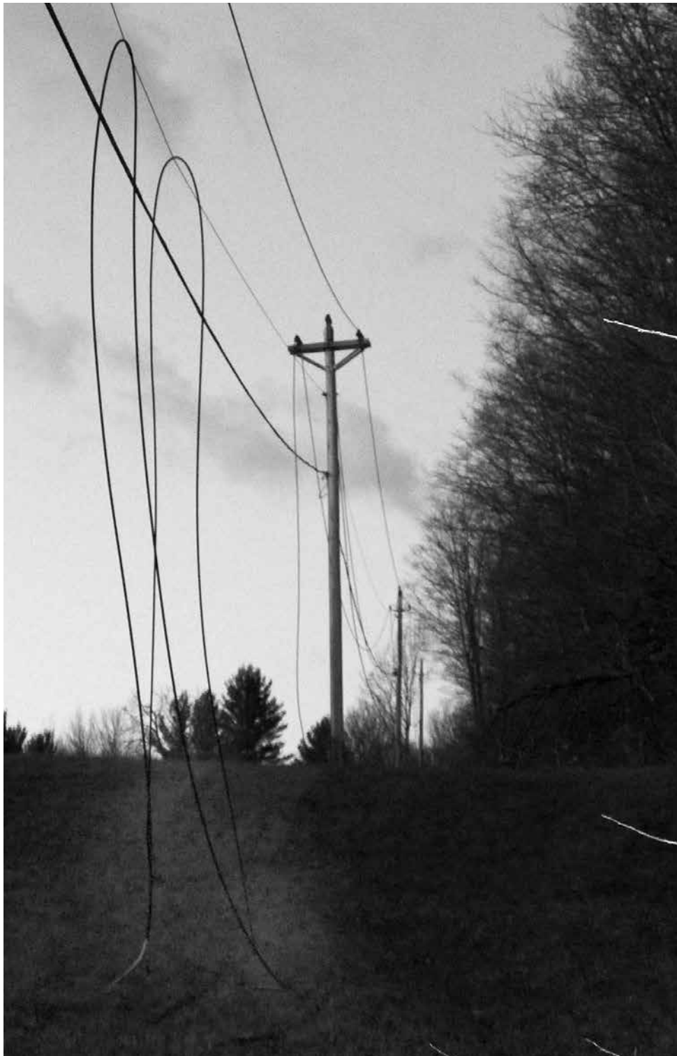
Loops of wire hang dangerously from this distribution line.
