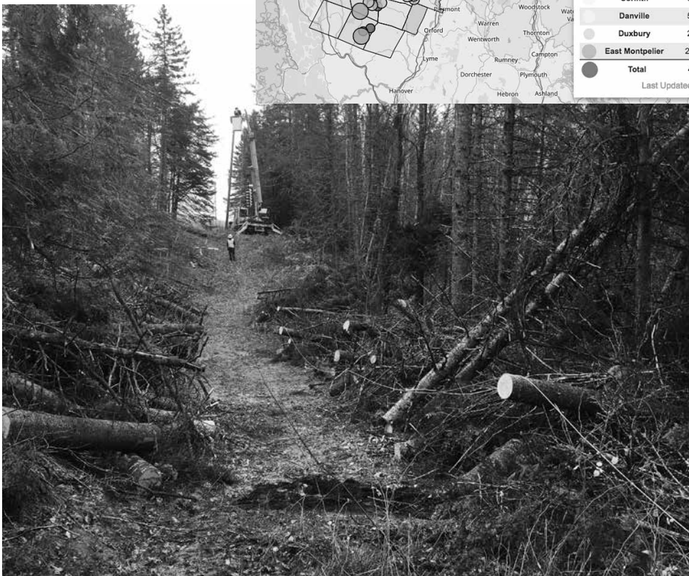
Crews work to repair a line in Fayston. The Right of Way is neatly lined with tree debris, all of which came down during the Halloween storm and had to be cleaned up as part of the restoration work.
