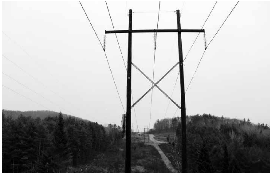
A VELCO transmission line. These high-voltage lines transmit up to 345,000 volts of electricity to utilities across the state, connecting with distribution utilities—like WEC—at substations. When a tree fell on a transmission line on December 14, it knocked out power to two WEC substations and more than 4,000 of WEC's members.
