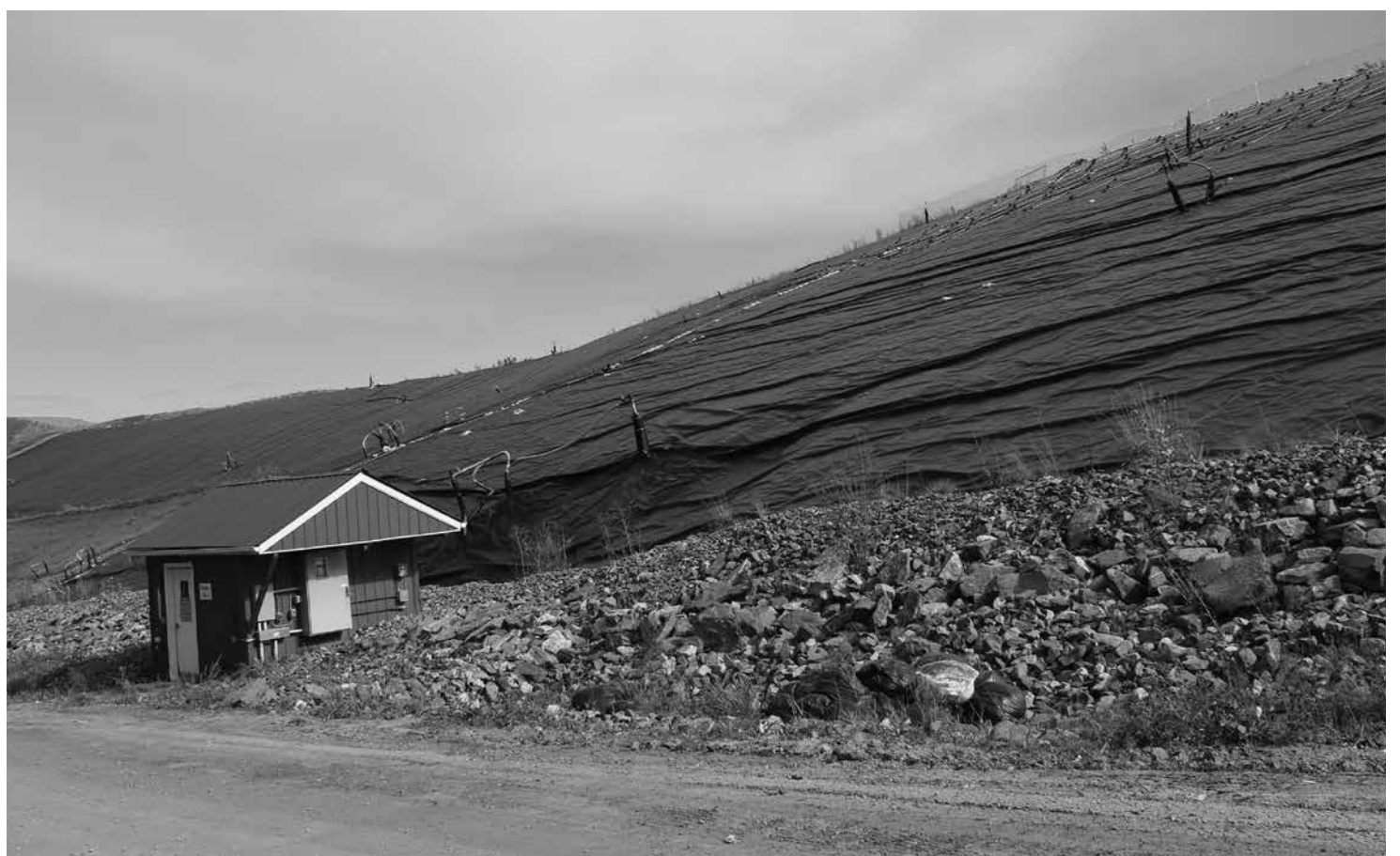
A capped section of the Coventry landfill. Methane produced by anaerobic activity in the landfill powers WEC's landfill-gas-to-electricity plant. The landfill expansion temporarily disrupted this process, reducing the plant's output in 2021.
