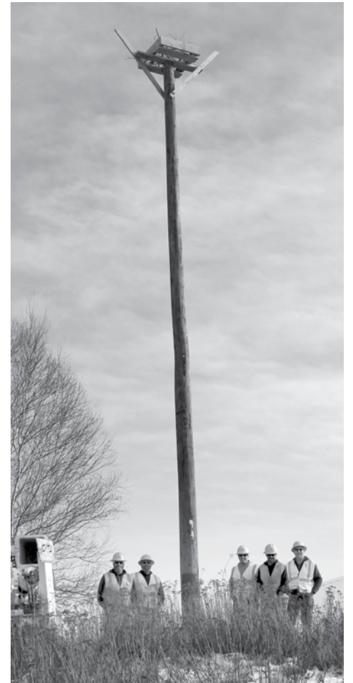
Members of WEC's operations team built a platform on a 40-foot pole on the highest point of a hill in Coventry across from the landfill and WEC's landfill gas-to-electricity generation plant. The new platform is intended to attract nesting osprey away from their first choice – an H-frame transmission pole.
