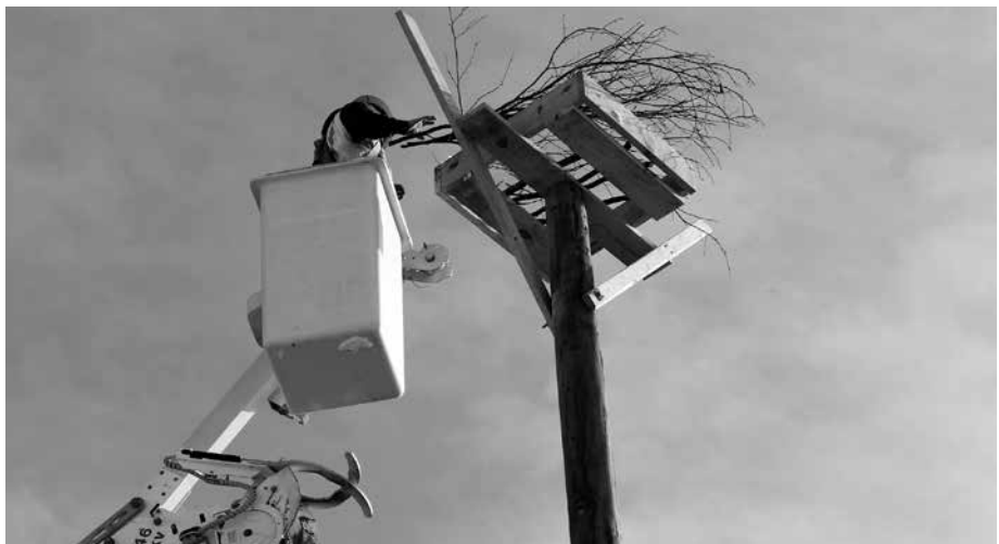
Summoning his inner raptor, Amos Turner arranges sticks on a platform high in the sky to entice osprey to build a nest there – instead of on an H-frame carrying transmission lines from WEC’s landfill gas-to-electricity generation plant in Coventry. Learn about WEC’s osprey relocation project on page 8.
